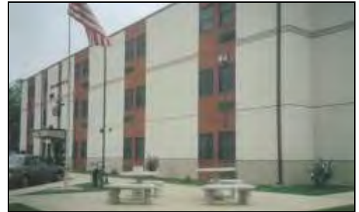
Cabell-Huntington Unity Apartments
