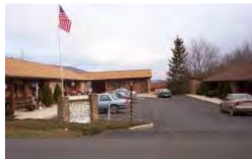
Beth Place Apartments
